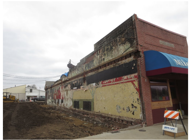
The wall that saved the old 'Chink's' building from fire loss
